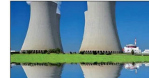
Nuclear Power : pipeline system, nuclear island lubrication system and conventional island wastewater treatment
